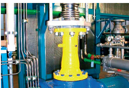
Gas turbine installation
